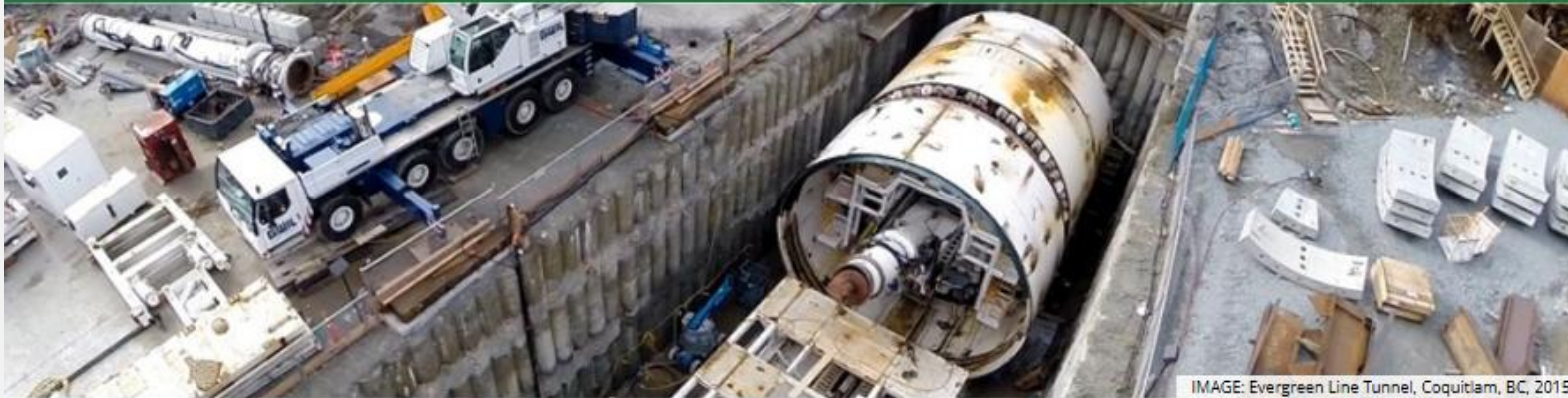
IMAGE: Evergreen Line Tunnel, Coquitlam, BC, 2015
